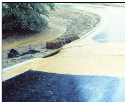
Stormwater discharge into a sewer.
