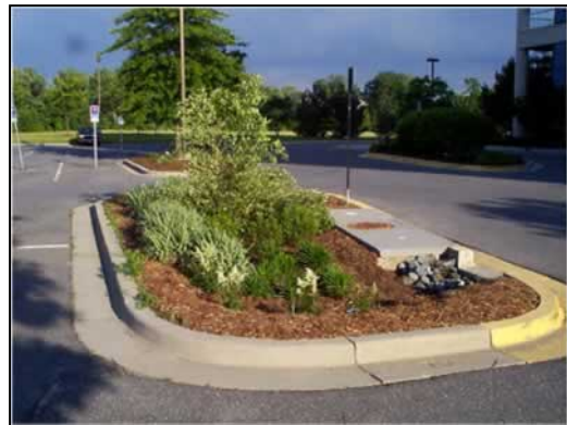
Low impact development: Bioretention area.
